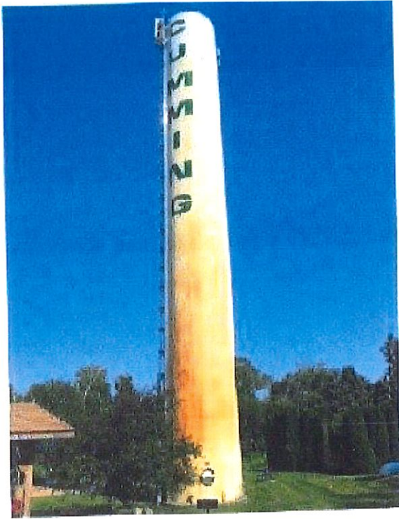
84,000 GALLON STANDPIPE TANK
